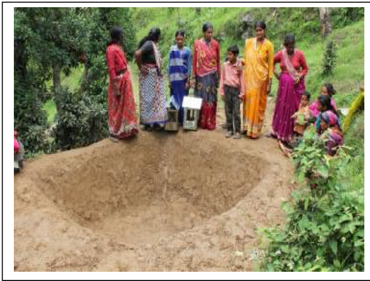
Installing a polythene-lined water tank at Lamudiyar village, district Almora.
