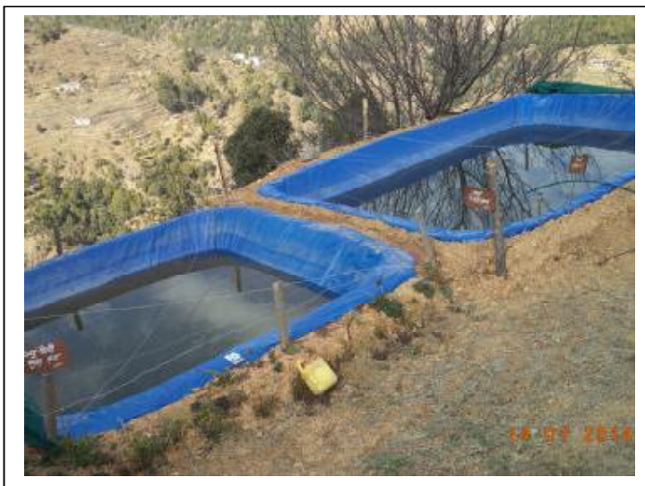
Polythene-lined water tanks at village Galla, district Nainital. Water from these tanks is used for the purpose of raising apple and peach saplings in the village nursery.
