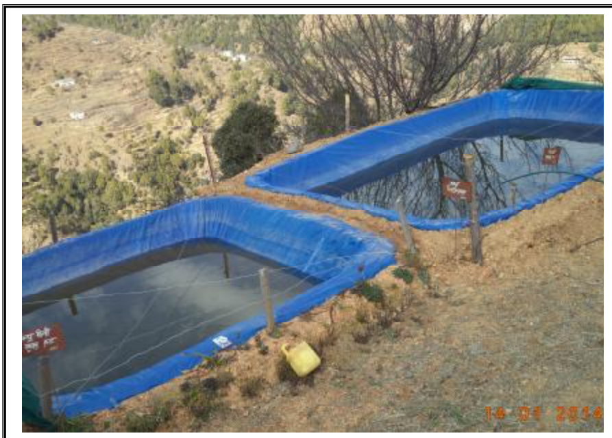
Polythene lined water tanks at Galla village, district Nainital.
