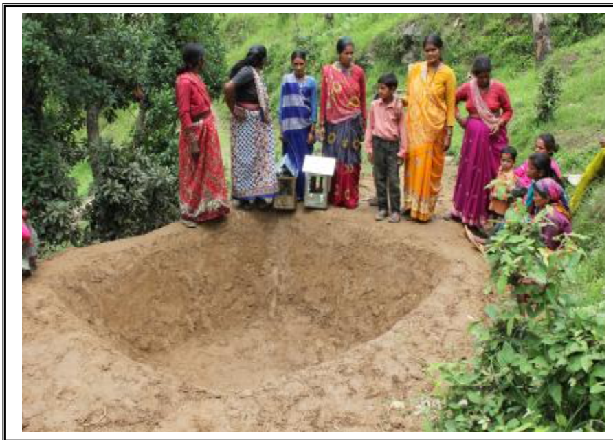
Installing a polythene lined water tank at Lamudiyar village, district Almora.
