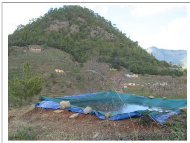
A polythene-lined water tank at Galla, district Nainital. The village experiences acute shortage of water during the summers. The tanks have proven very useful to the community.
